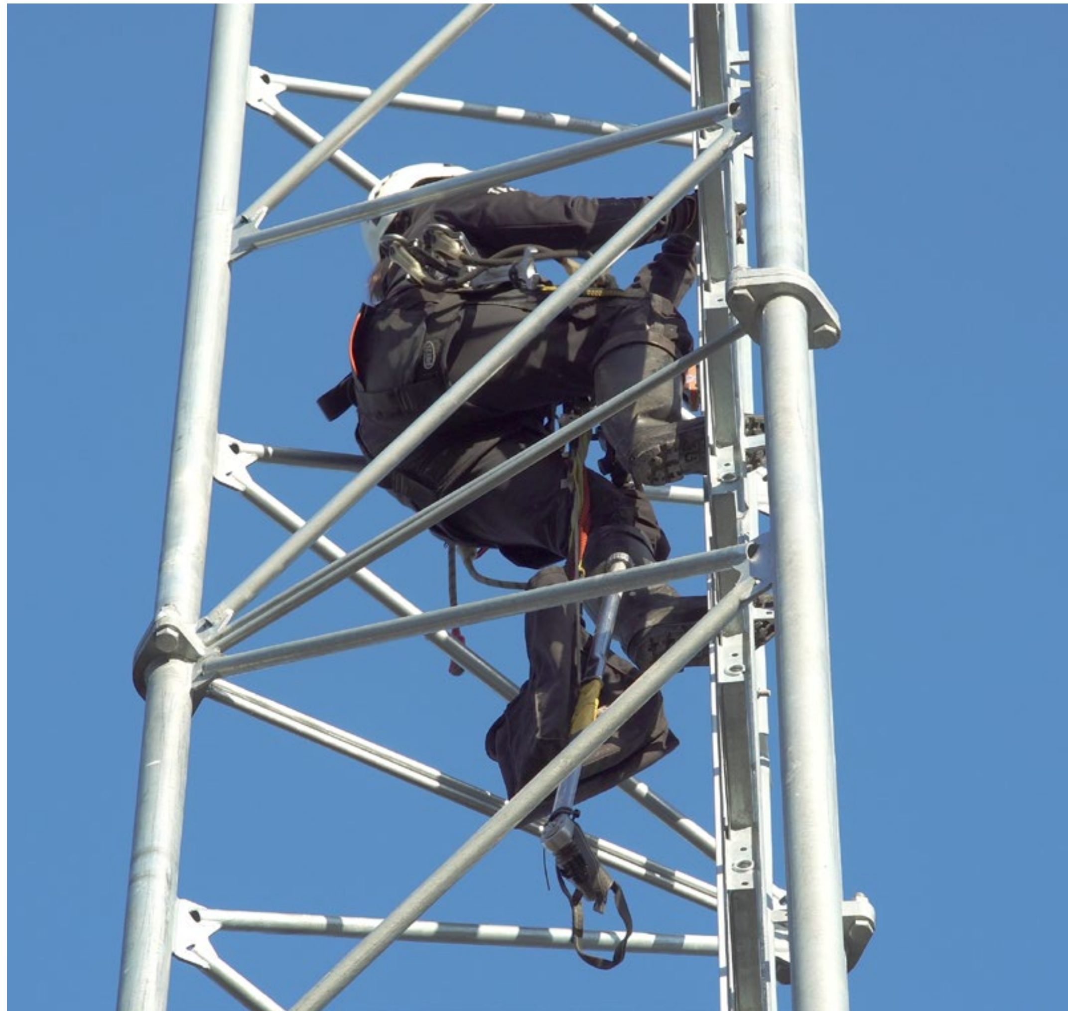
Tools and tool bags hang between a technician's legs when climbing a mast.
