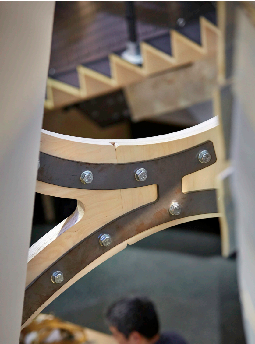
Integrated seating and work surfaces comprise the outside-facing perimeter of the Treehouse. Structural connections are exposed throughout.
